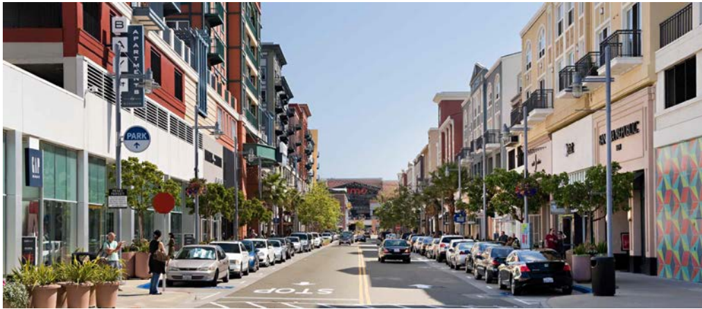
Bay Street, residential over retail
